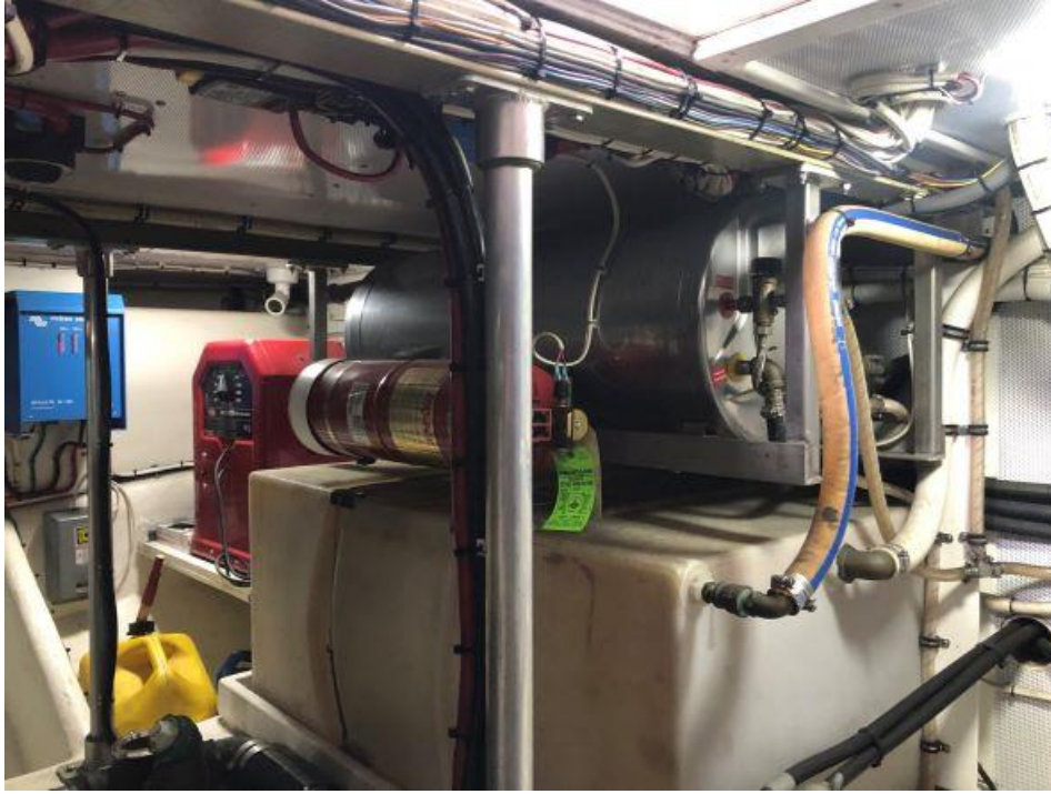
3. Forward engine room. Hot water heater and potable water tank.
