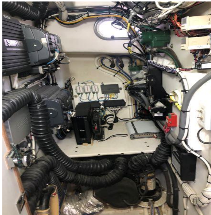
8. Electronics and gear locker, forward of pilothouse.
